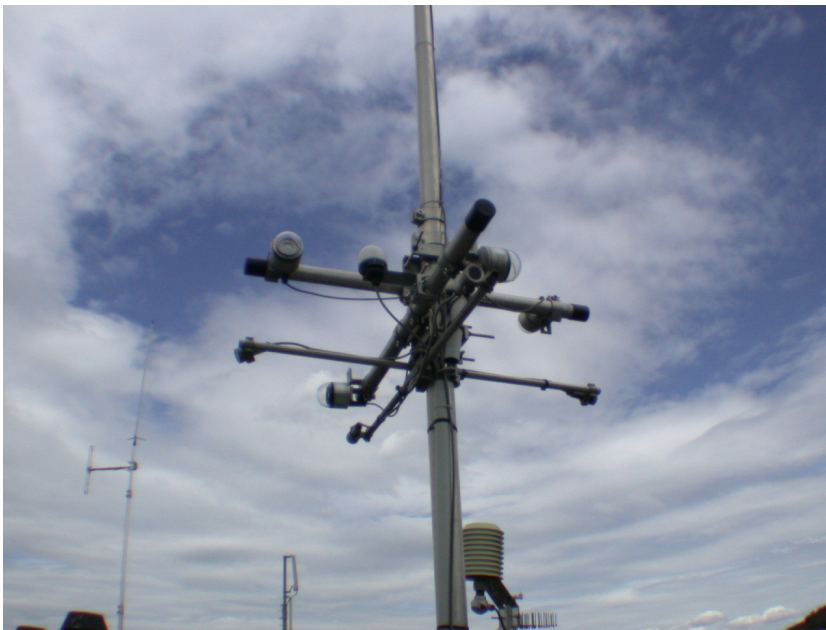
Figure 57: Antenna carrying vertical irradiance and illuminance sensors.
